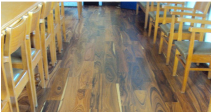
Santa Maria de Lamas Parish Council: 220 m 2 of glue-down Corkcomfort Pebbles Fog and 168 m 2 of floating Woodcomfort Palisandro Santos.
